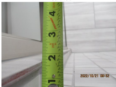
Shower curb "step-down" should be a minimum of 2"
