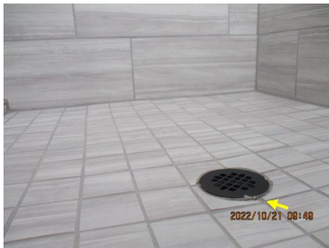
Drain is raised above the tile at the master shower
