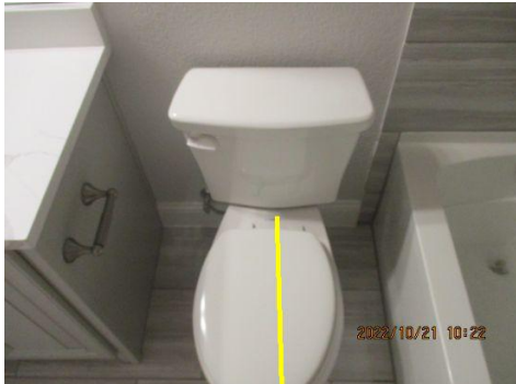
Commode is mounted crooked on the floor
