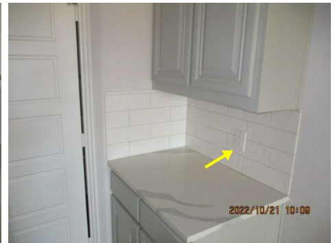
Missing or damaged receptacle, switch or junction box covers ~ Damaged
