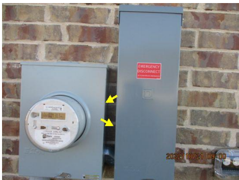
Missing Caulk observed. The exterior of home should be re-caulked to prevent water penetration.
