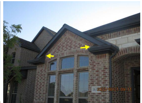
Missing flashing observed
