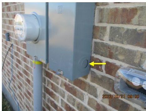
Knockout should be sealed to prevent water penetration
