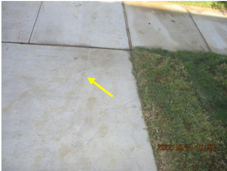
Cracks and damage observed at driveway
