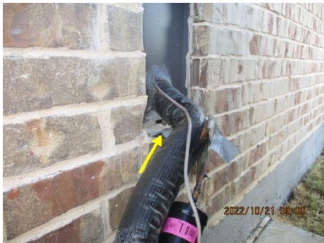
Re-Point (Repair/patch) missing or cracked mortar
