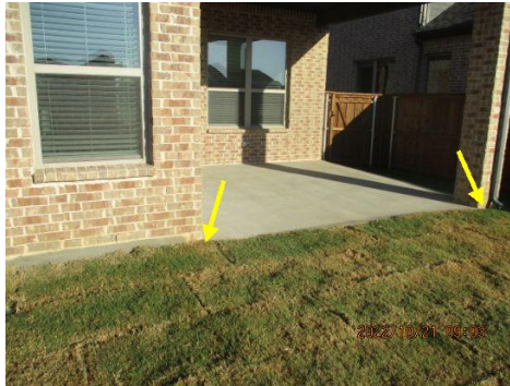
Improper or inadequate grading around the foundation Soil level should be at least 4" below brick/stone siding
