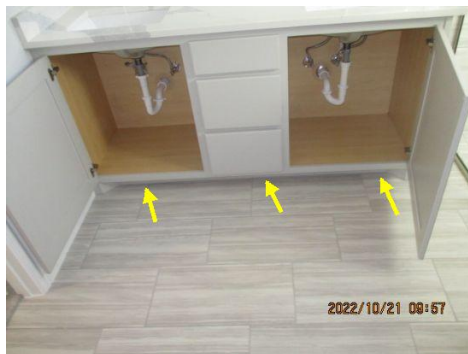
Missing/cracked grout observed at flooring. Repair/replace as necessary. ~ Master bathroom
