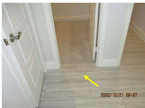
Tiles on floors are "hollow", missing thin-set cement. These tiles are more prone to cracking. ~ Master bathroom
