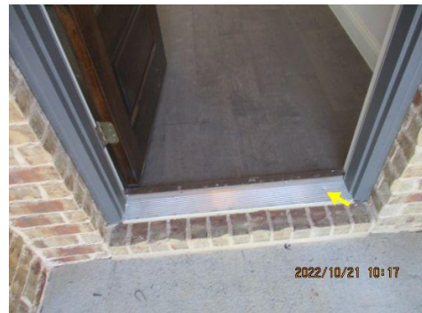
Damaged/dented threshold observed
