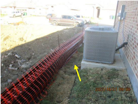
Water ponding observed – Grading should be improved
