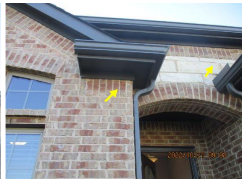
Re-Point (Repair/patch) missing or cracked mortar
