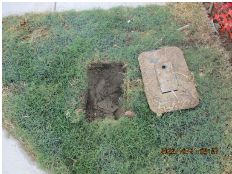
Meter box full of dirt, meter not visible to check for active leaks on the supply side of plumbing
