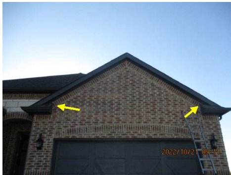
Missing flashing observed
