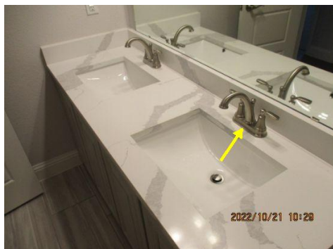
Fixtures are not securely mounted ~ Guest bathroom
