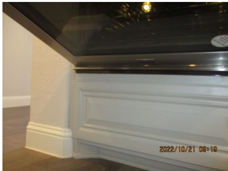
Door "hits" the trim when opening oven door
