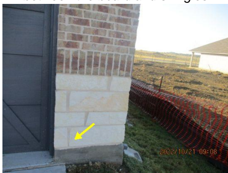
Weep holes are not present at lower part of masonry/stone wall. The weep holes allow any water absorbed by the masonry/stone wall to drain out
