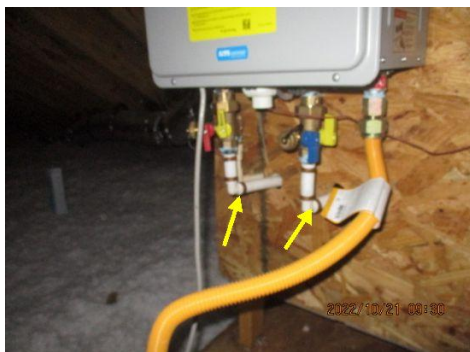
Plumbing supply lines should be insulated
