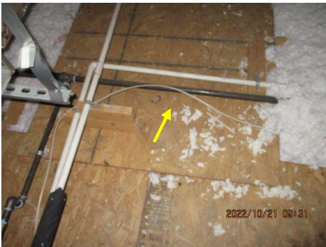
Unprotected wiring observed in the attic walkway
