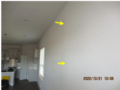
Bow or wave in the wall observed ~ Living room, SW bedroom
