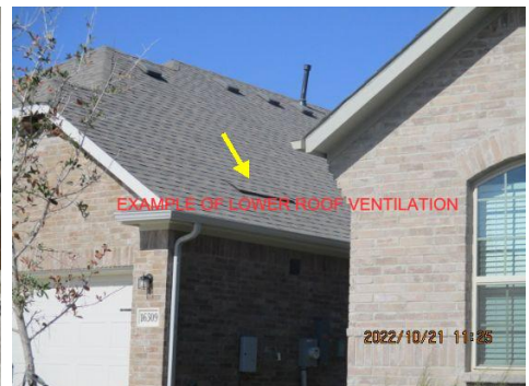
Missing soffit or lower roof intake ventilation. Baffles installed in the attic as required for this type of ventilation
