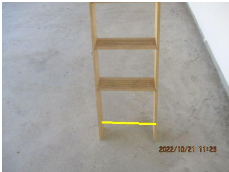
Missing step observed
