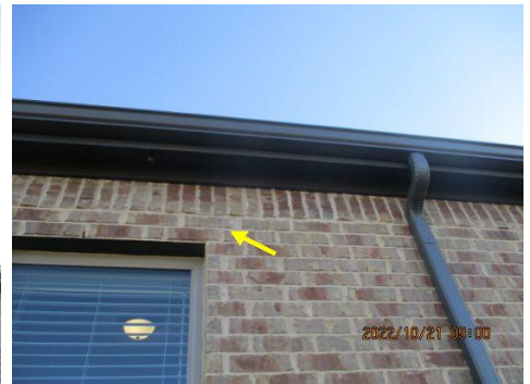
Re-Point (Repair/patch) missing or cracked mortar
