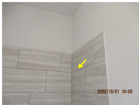
Missing caulk/grout at tubs and showers. Recommend re-caulking and/or /replacing grout to prevent water penetration
