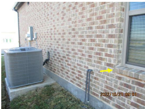
Re-Point (Repair/patch) missing or cracked mortar
