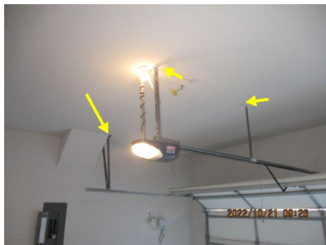
Holes in ceiling should be sealed for proper fire-blocking in garage
