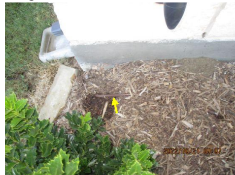
Drip line should be buried to prevent damage
