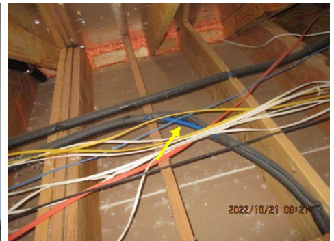
Plumbing supply lines should be insulated
