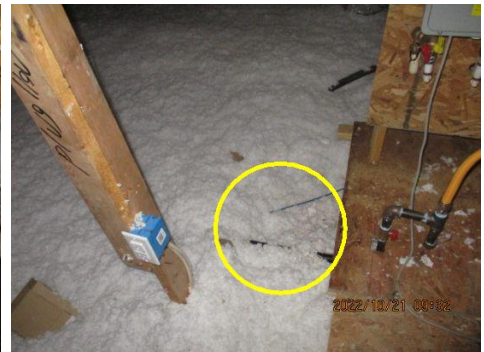
Uneven insulation observed
