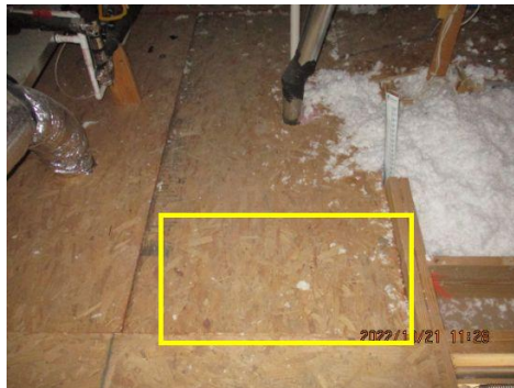
Attic walkway is not adequately supported. Decking moves up/down when walked upon
