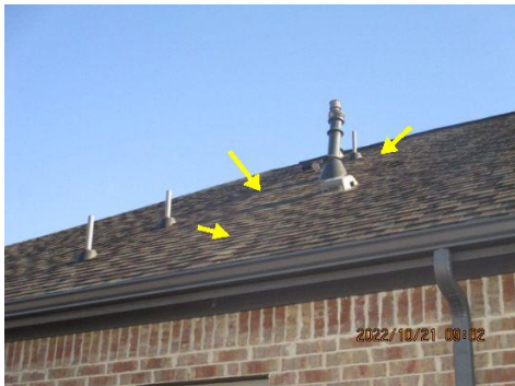
Irregular, "wavy" surface observed
