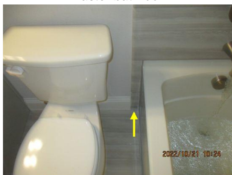
Missing/cracked grout observed at flooring. Repair/replace as necessary. ~ Guest bathroom
