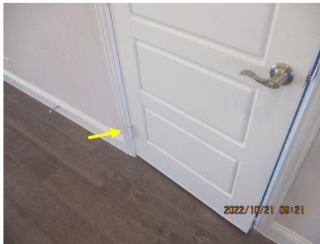
Garage entry door does not close completely with self-closing hinge or automatic closing device
