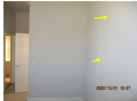
Bow or wave in the wall observed ~ Living room, SW bedroom
