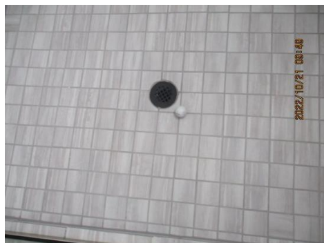
Shower pan is not sloped toward the drain, possible standing water
