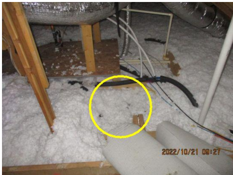
Uneven insulation observed
