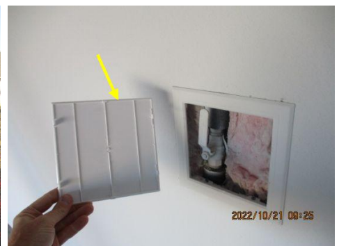
The water shutoff valve box is plastic. A fire-rated box is required at this location. I was not able to verify if this plastic box is fire-rated.
