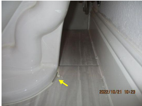
Commode is missing caulking ~ Guest bathroom
