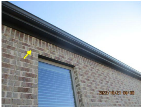
Re-Point (Repair/patch) missing or cracked mortar
