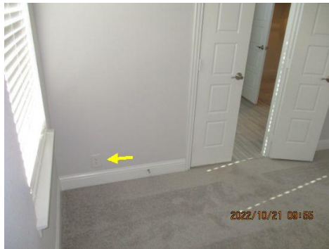
Receptacle is not secured in place, loose on the wall ~ Master
