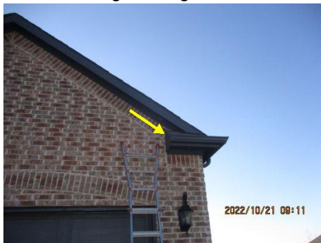
There are nail heads or staples exposed (missing sealant) on flashing(s), roof vents and in the cap shingles. Recommend sealing to prevent water penetration.
