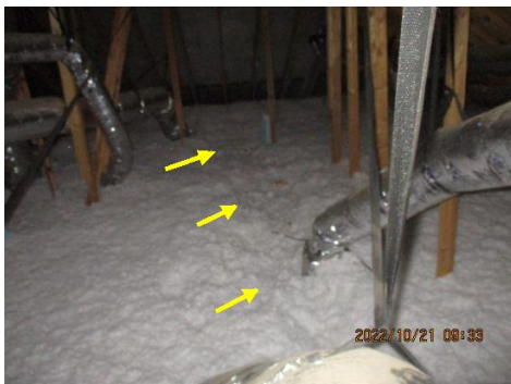
Uneven insulation observed
