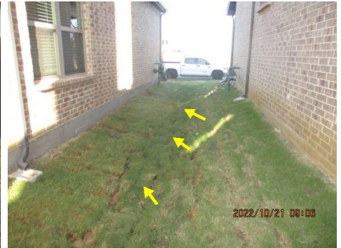
Water ponding observed – Grading should be improved
