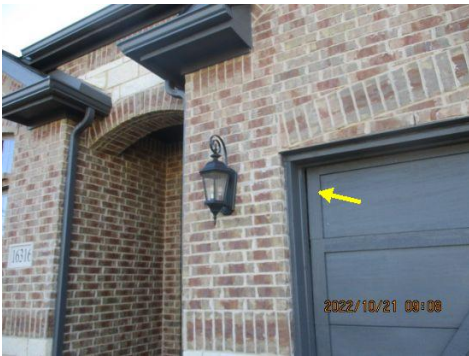
Overhead door is not square in the door opening
