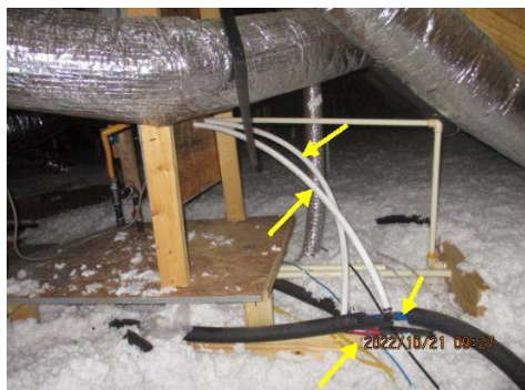
Plumbing supply lines should be insulated
