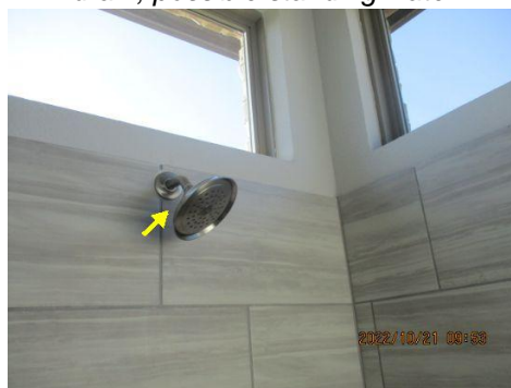
Fixtures are not securely mounted ~ Master shower
