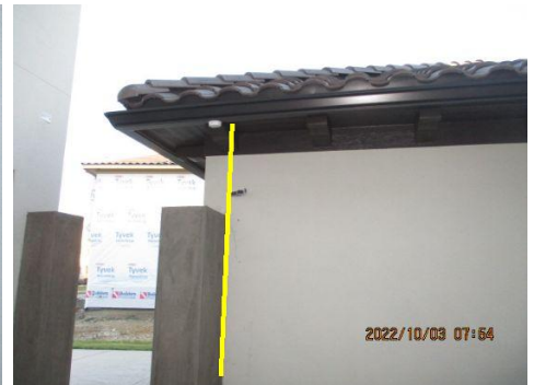
Missing down spouts observed
