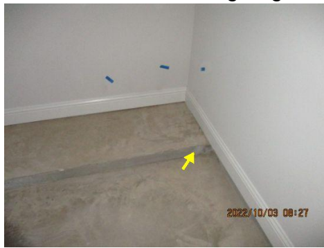
Chipped concrete observed ~ 1- car garage
