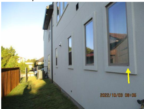
Missing drain cover(s) at window(s)
