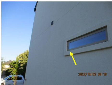
Missing drain cover(s) at window(s)
