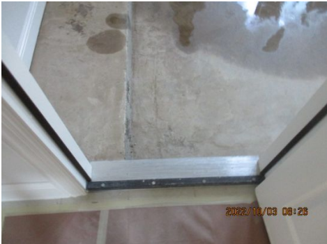
Loose/unsupported threshold observed ~ 1- car garage entry
