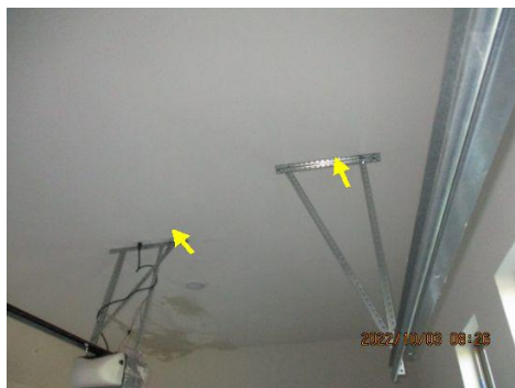
Holes in ceiling should be sealed for proper fire-blocking in garage ~ 1- car garage
