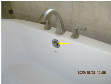
Missing handle at master tub drain stop operator
