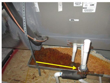
Safety pan is not tilted toward the drain ~ Unit 3
