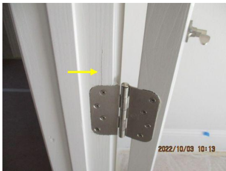
Cracked door or door frame observed ~ Master bathroom
