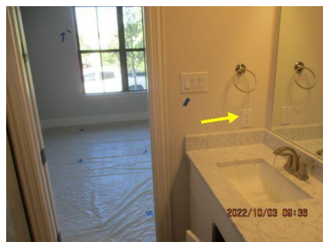
Receptacle is not secured in place, loose on the wall ~ Lower SW bathroom
