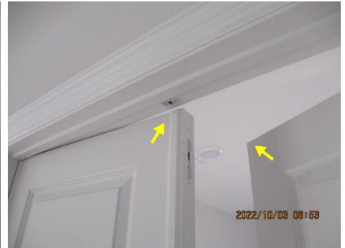
Door out of square and drags/binds on the frame or other door ~ Media room
