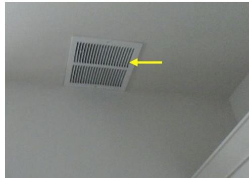
Missing filter at make-up air vent
