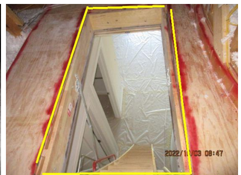
Missing/loose insulation observed
