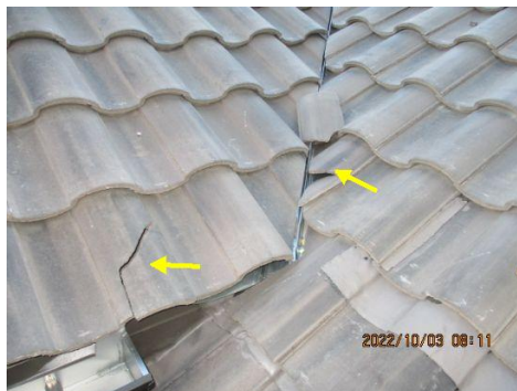
Cracked tiles observed ~ Above courtyard
