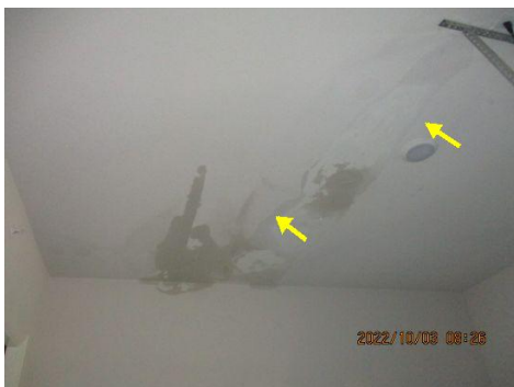
Ceiling water stains observed ~ 1- car garage
