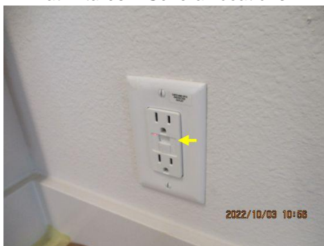
GFCI button stays depressed when reset ~ Master bathroom
