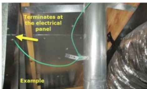
Bonding or grounding - Appliances such as water heaters, furnaces, chimneys and electrical gutters do not have proper bonding ~ See page 2 for additional information
