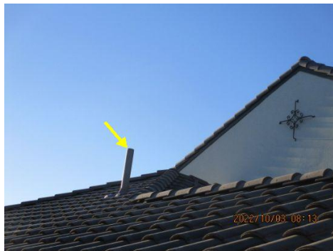
Missing cap at roof vent pipe
