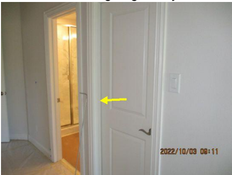
Door binds on the hinge side of frame, difficult to close. ~ Upper SW bedroom closet
