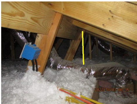
Missing/damaged support strap for duct work. Ducting should be supported above insulation ~ Garage attic
