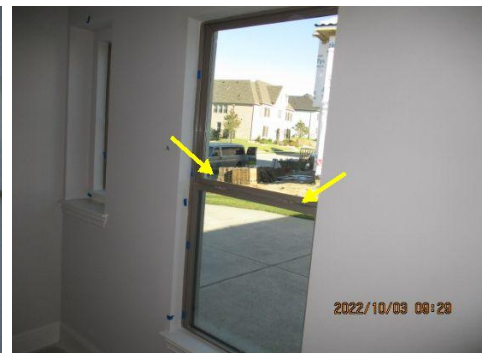
Tilt out latch do not operate properly ~Study
