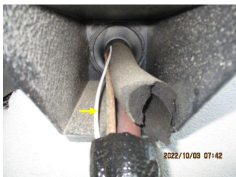
Missing/damaged/loose insulation on refrigerant pipe(s)
