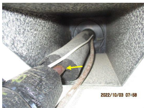
Missing/damaged/loose insulation on refrigerant pipe(s)
