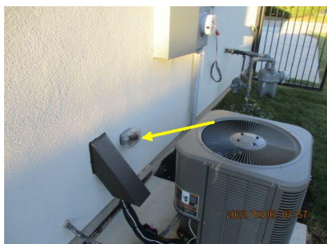
GFCI protection missing at: Outdoor receptacles
