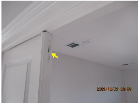
Door latch does not operate ~ Media room
