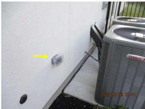
Receptacle is not secured in place, loose on the wall
