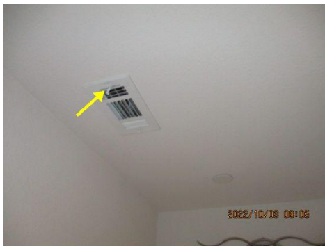
Register does not open close completely ~ Upper SE bathroom
