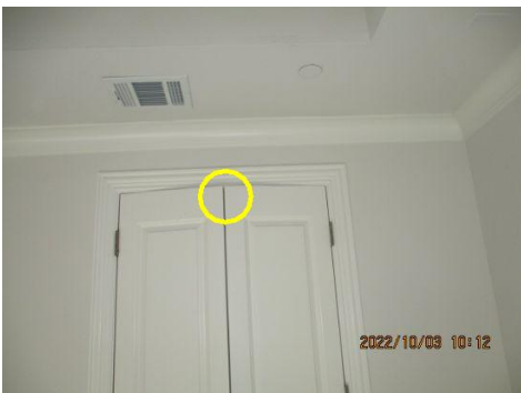
Door out of square and drags/binds on the frame or other door ~ Master bathroom
