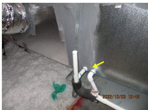
Missing or cracked tape/mastic observed at the air handler. I recommend resealing mastic/tape to prevent heat/air from blowing out ~ Unit 3
