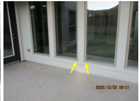
Missing drain cover(s) at window(s)
