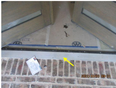
Loose/unsupported threshold observed ~ Front door
