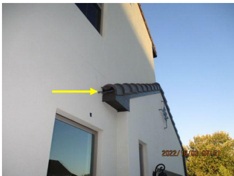
Missing kick-out flashing observed
