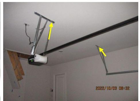
Holes in ceiling should be sealed for proper fire-blocking in garage ~ 2- car garage
