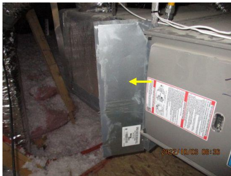
Filter door is not insulated ~ All 3 units
