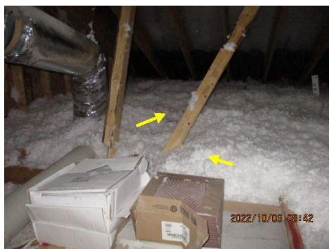
Uneven insulation observed ~ Upper attic
