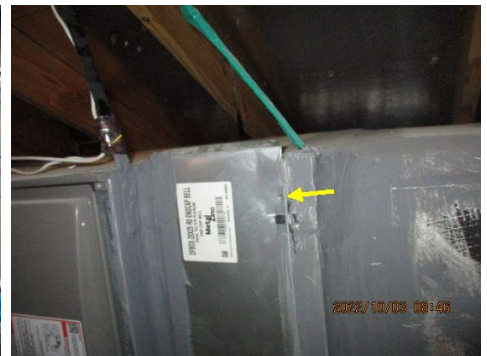
Holes observed in filter doors ~ Units 2 and 3
