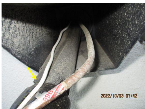
Missing/damaged/loose insulation on refrigerant pipe(s)
