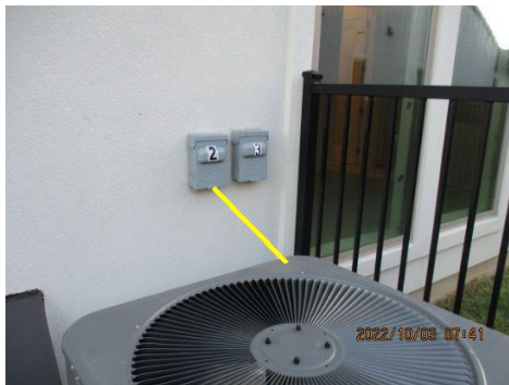
Inadequate access to disconnect switches an A/C condenser(s). A minimum of 36 inches of clearance in front of and 30 inches beside the disconnect switches is required
