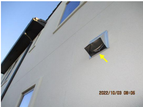
Damper does not close completely
