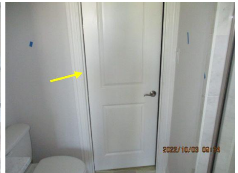
Door binds on the hinge side of frame, difficult to close. ~ Lower SW bedroom closet
