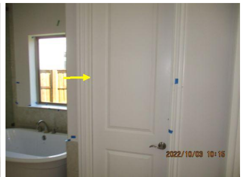
Door binds on the hinge side of frame, difficult to close. ~ Master water closet
