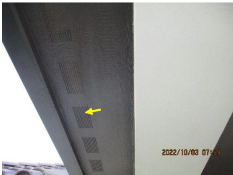
Damaged soffit vent observed ~ Above rear patio
