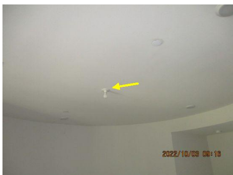
Missing protective globe around bulbs at fixtures ~ Several locations
