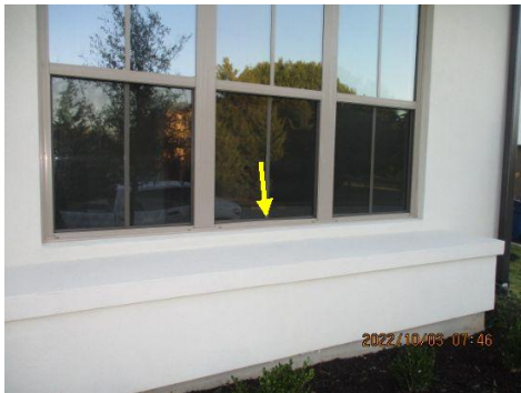
Window frame has a "bow" at the lower portion ~ SW bedroom
