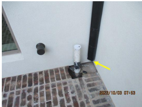
Missing down spouts observed ~ Courtyard - all locations
