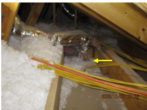
Missing/loose insulation observed ~ Garage attic
