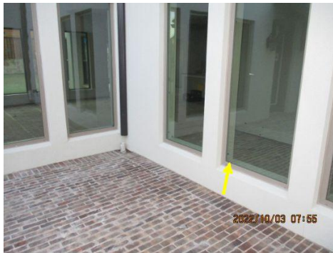
Missing drain cover(s) at window(s)
