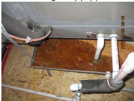
Safety pan contains water and is rusted ~ Unit 2
