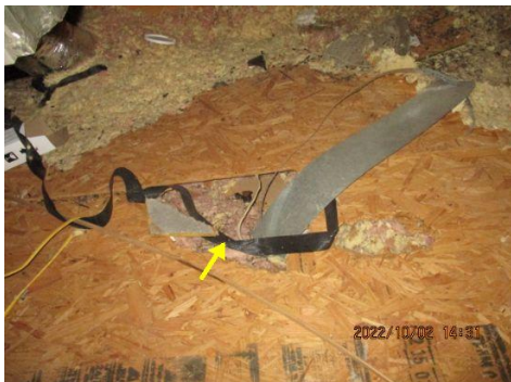
Missing/loose insulation observed
