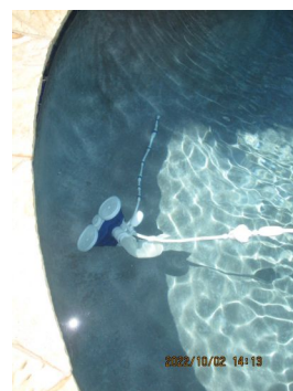
Pool sweep stopped operating after a few minutes. The pump sounded like it lost its prime.
