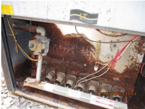
Pool heater is rusted/corroded
