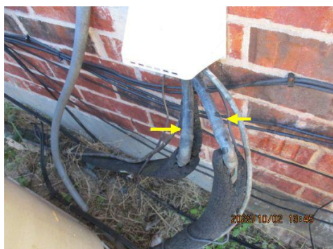
Missing/damaged/loose insulation on refrigerant pipe(s)
