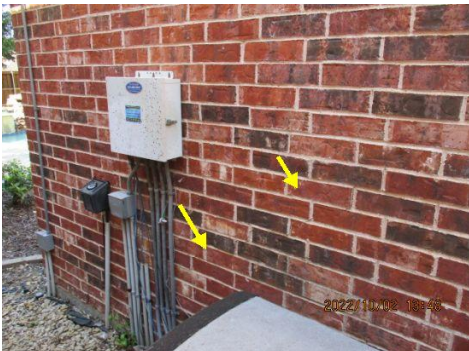
Re-Point (Repair/patch) missing or cracked mortar
