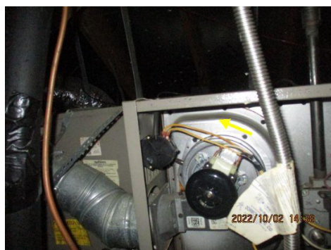
Missing or cracked tape/mastic observed at the air handler. I recommend resealing mastic/tape to prevent heat/air from blowing out ~ Unit 1
