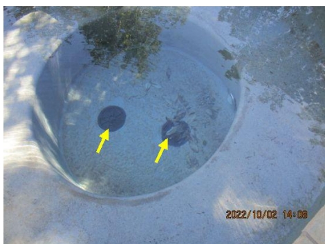
The presence of a blockable main drain (potential entrapment hazard) observed at the hot tub. I recommend the installation of an anti-vortex cover which is the current standard in the industry
