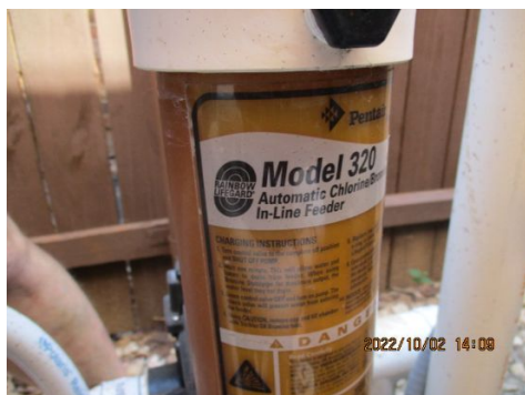
Inline chlorine feeder observed at pool equipment. I also observed a chlorine bucket(s) in the pool/spa. I recommend verifying the inline chlorine feeder is operating properly
