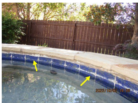
Efflorescence observed
