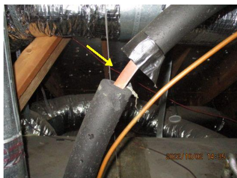
Missing/damaged/loose insulation on refrigerant pipe(s)
