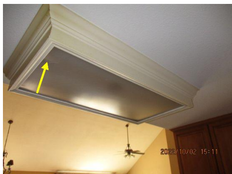
Kitchen light cover is cracked
