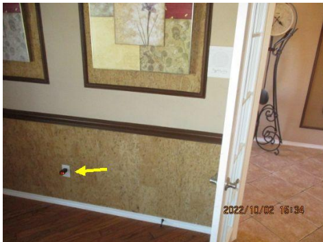
Difficult/unable to plug in testing device into receptacles ~ Study
