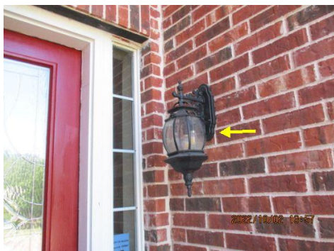
Fixtures installed upside down ~ Coach light, porch light
