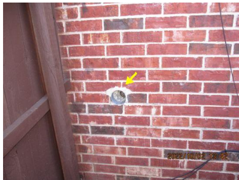
Missing cover at combustion air vent
