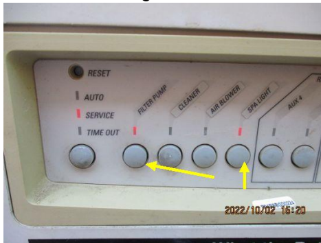
When I turn on the spa light, the pump comes on at the same time
