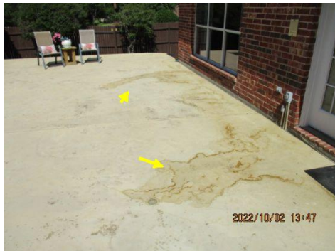
Water ponding/stains observed
