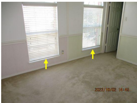
2nd story windows within 24" of the floor should be fixed (not openable) or have openings through which a 4 – inch diameter sphere cannot pass ~ Upper SE bedroom
