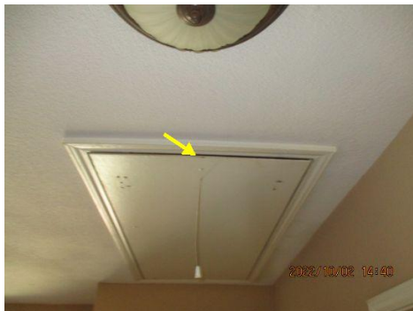
Attic access door does not close completely – Adjust as necessary
