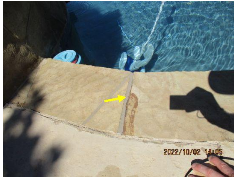
Re-point cracked/missing mortar at coping and/or tile to prevent water penetration
