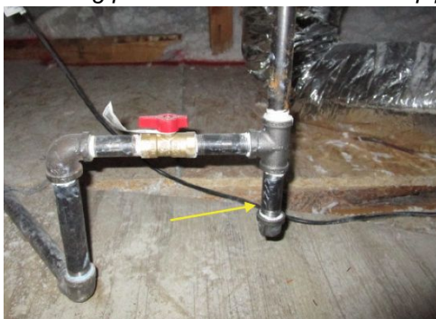
Gas line sediment traps are not present at the water heater(s) and heating system(s)
