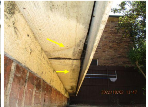
Deteriorated wood observed at siding and/or trim boards. Repair/replace as necessary.
