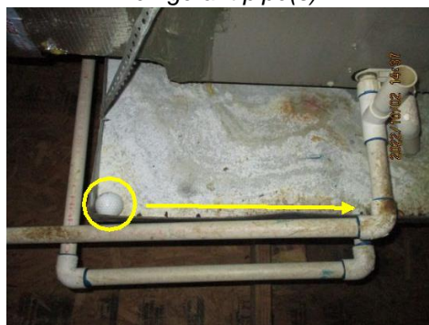
Safety pan is not tilted toward the drain ~ Unit 2
