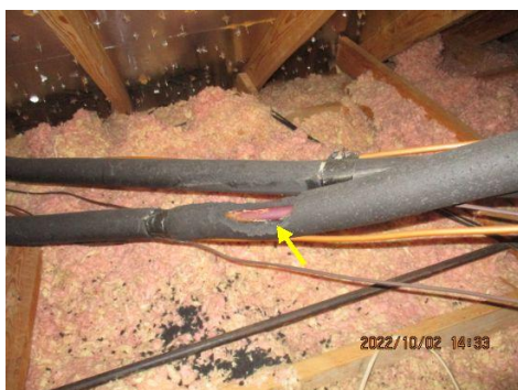
Missing/damaged/loose insulation on refrigerant pipe(s)
