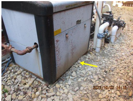
Heater should be raised 3" above the grade
