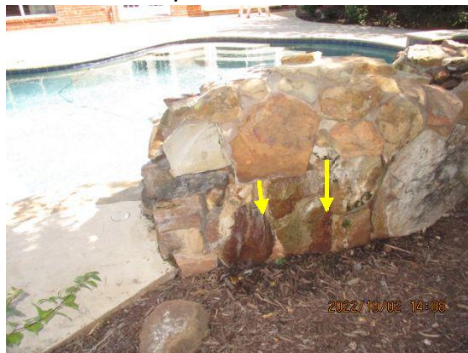
Waterfall is leaking water on the back side of the waterfall
