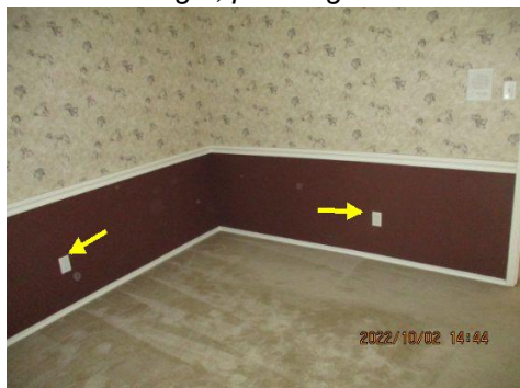
Difficult/unable to plug in testing device into receptacles ~ Upper SW bedroom
