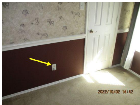
Burn mark observed the receptacle ~ Upper SW bedroom
