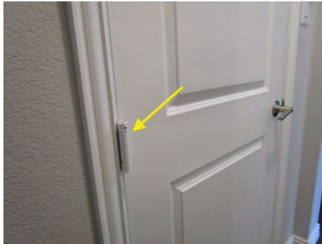
Garage entry door is not equipped with a self-closing hinge or automatic closing device
