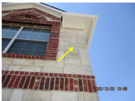
Re-Point (Repair/patch) missing or cracked mortar
