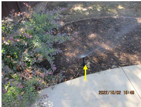
Leaks/broken heads observed at zone(s): 5
