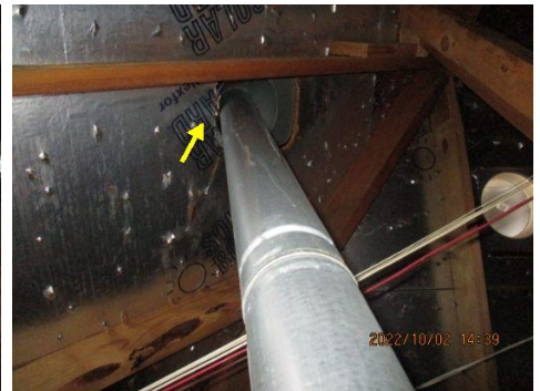
Vent pipe too close to combustible materials, a minimum 1" clearance is required
