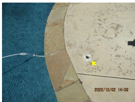
Damaged/missing cap observed
