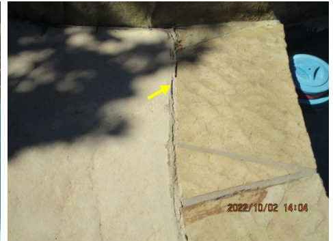
Missing/deteriorated mastic observed. Mastic should be resealed between the deck and coping to prevent water penetration
