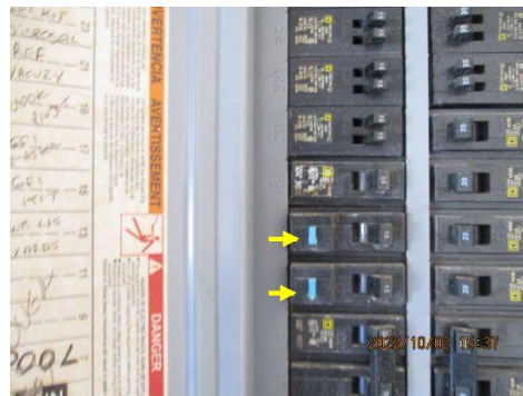
Arc-fault circuit breaker(s) did not trip when tested with self-test button
