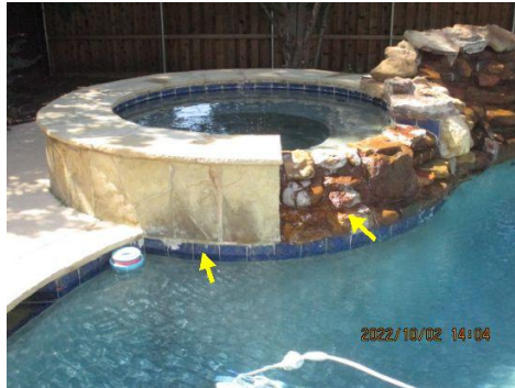
Efflorescence observed
