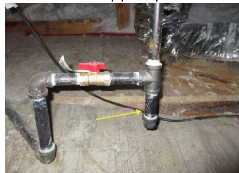
Gas line sediment traps are not present at the pool/spa heater
