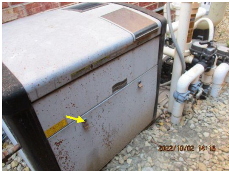
Heater latch is damaged, does not secure the cover in place
