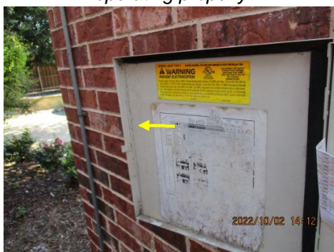
Missing weather stripping at control/timer box
