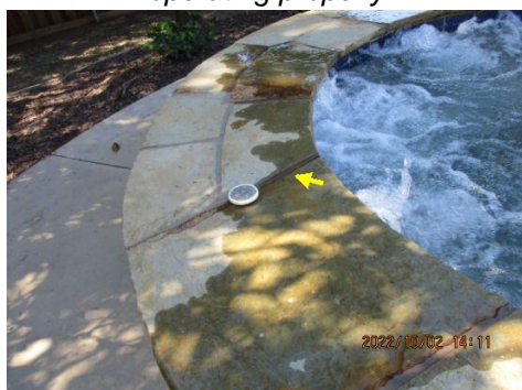
Uneven coping observed at hot tub
