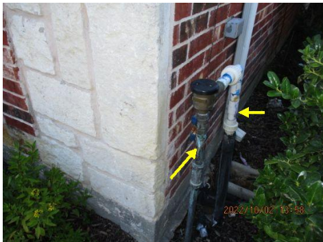
Backflow prevention device (double-check valve) should be insulated
