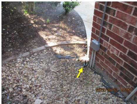
No water flow present at sprinkler head in zone(s):7
