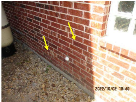
Re-Point (Repair/patch) missing or cracked mortar
