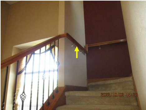
Handrail is loose on the wall
