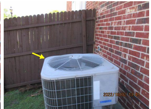
Condenser pad should be leveled for proper condenser operation
