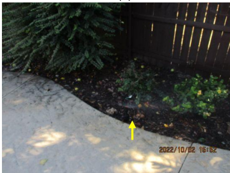
Leaks/broken heads observed at zone(s): 7
