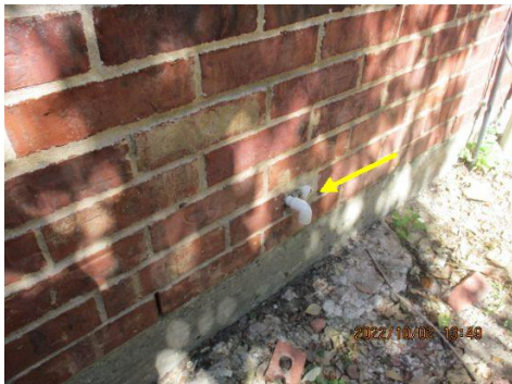
Discharge pipe is missing 90° elbow toward the ground
