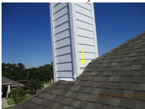
Cracked/damaged/loose siding observed. Replace/repair as necessary.
