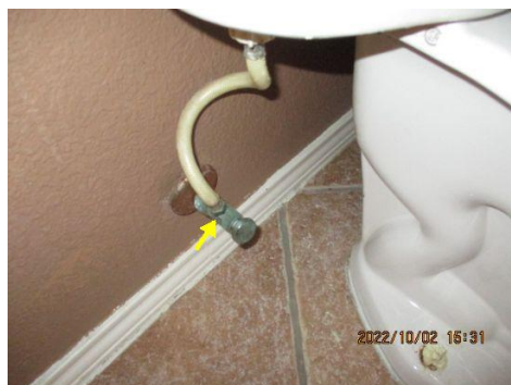
Corrosion observed at shutoff valves
