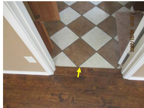
Missing transitions at wood flooring ~ Master bedroom
