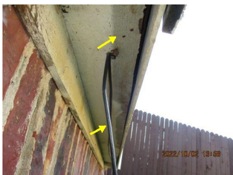
Deteriorated wood observed at siding and/or trim boards. Repair/replace as necessary.
