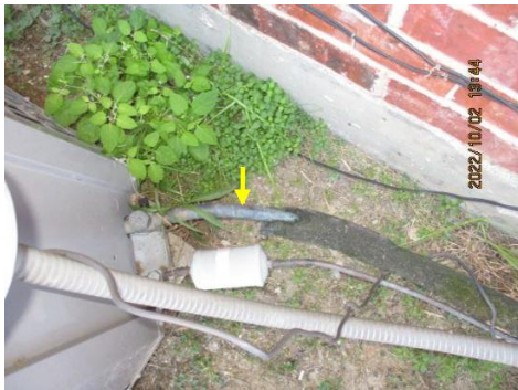
Missing/damaged/loose insulation on refrigerant pipe(s)
