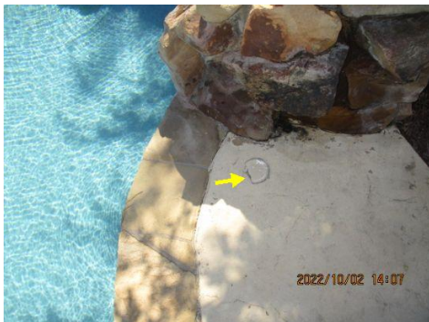
Damaged/missing cap observed
