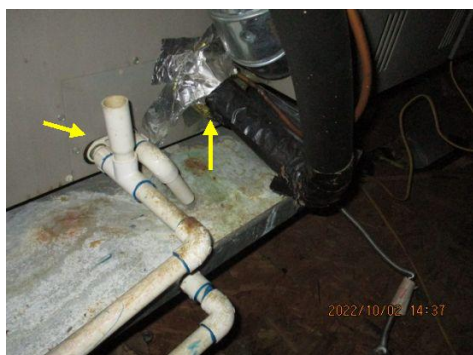
Missing or cracked tape/mastic observed at the air handler. I recommend resealing mastic/tape to prevent heat/air from blowing out ~ Unit 2
