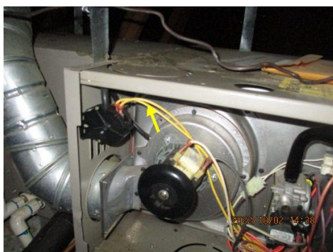
Missing or cracked tape/mastic observed at the air handler. I recommend resealing mastic/tape to prevent heat/air from blowing out ~ Unit 2
