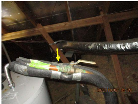
Corroded fittings or tank(s) observed
