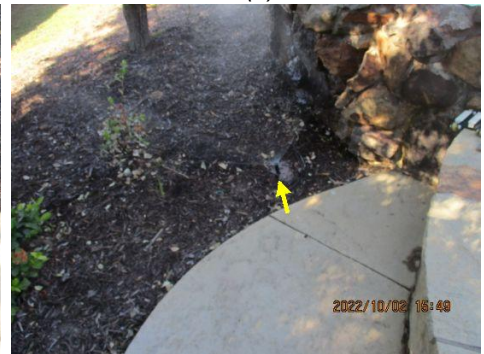
Leaks/broken heads observed at zone(s): 5
