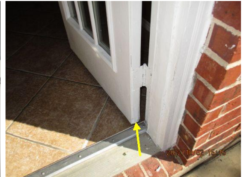
Patio door is water damaged
