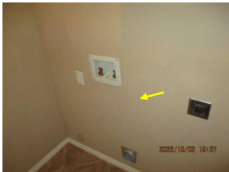
Water stains observed on interior walls ~ Laundry
