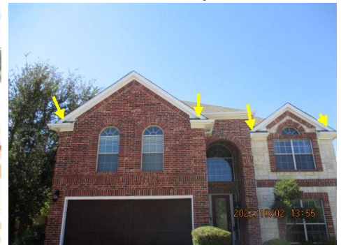
Fascia/trim boards in contact with shingles. Fascia/trim boards should have a gap to allow water to drain between the board and shingles.
