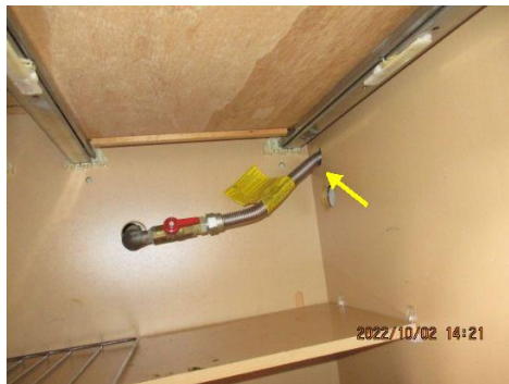
Gas appliance connectors should not pass through a cabinet wall. A Black iron pipe required at this location.
