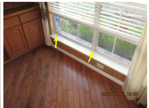
Water damaged /warped wood observed at sill ~ Study
