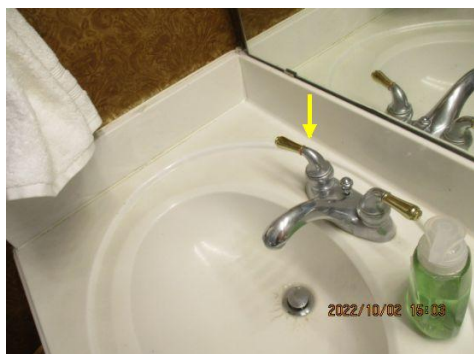
Faucet handle is loose ~ Master, powder bathroom
