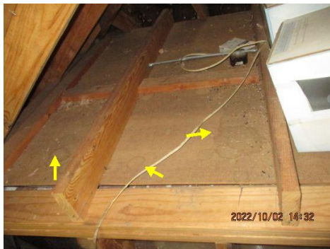
Evidence of water penetration, water stains observed
