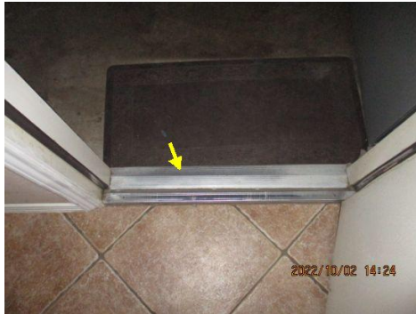
Loose/unsupported threshold observed ~ Garage entry door
